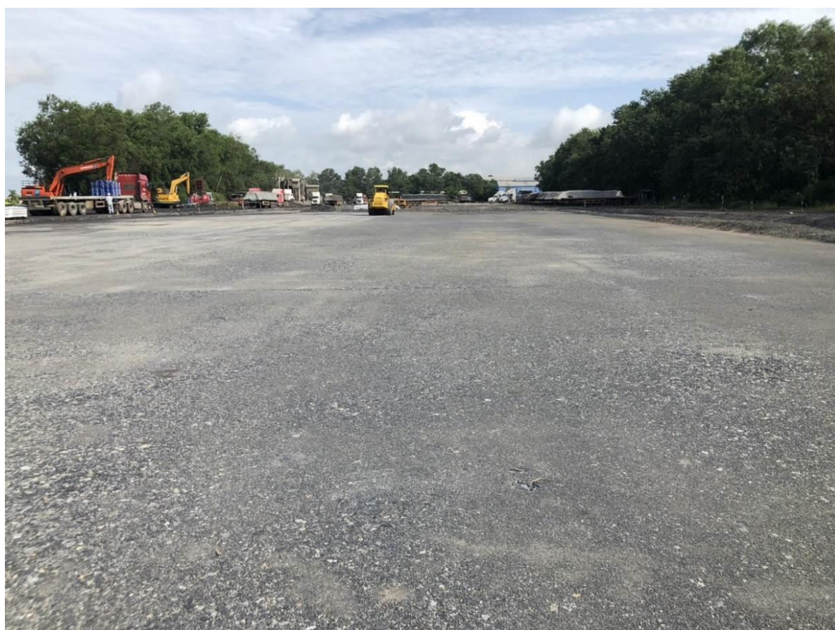
INFRASTRUCTURE OF BEN KEO JETTY – FICO YTL - TAY NINH
